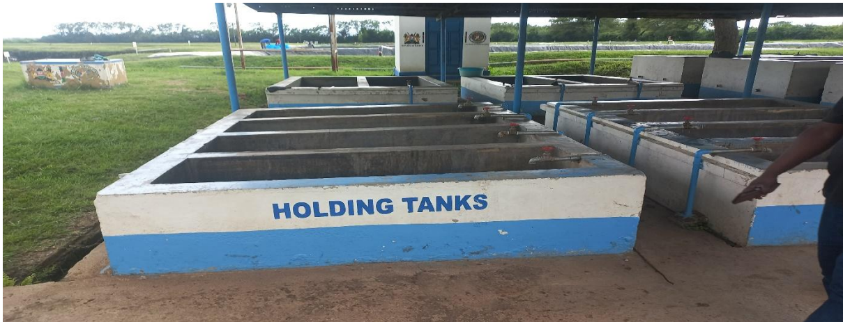
Plate 18: Holding tanks in the training facility
