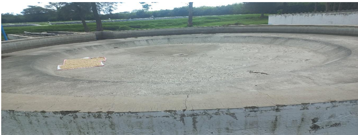
Plate 19: A concrete tank for holding fries at the training facility
